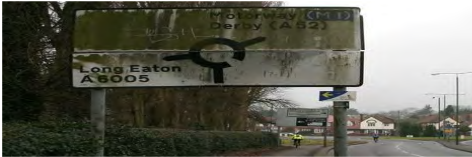
Figure 2.8 Example of a Bad Condition of Road Sign
