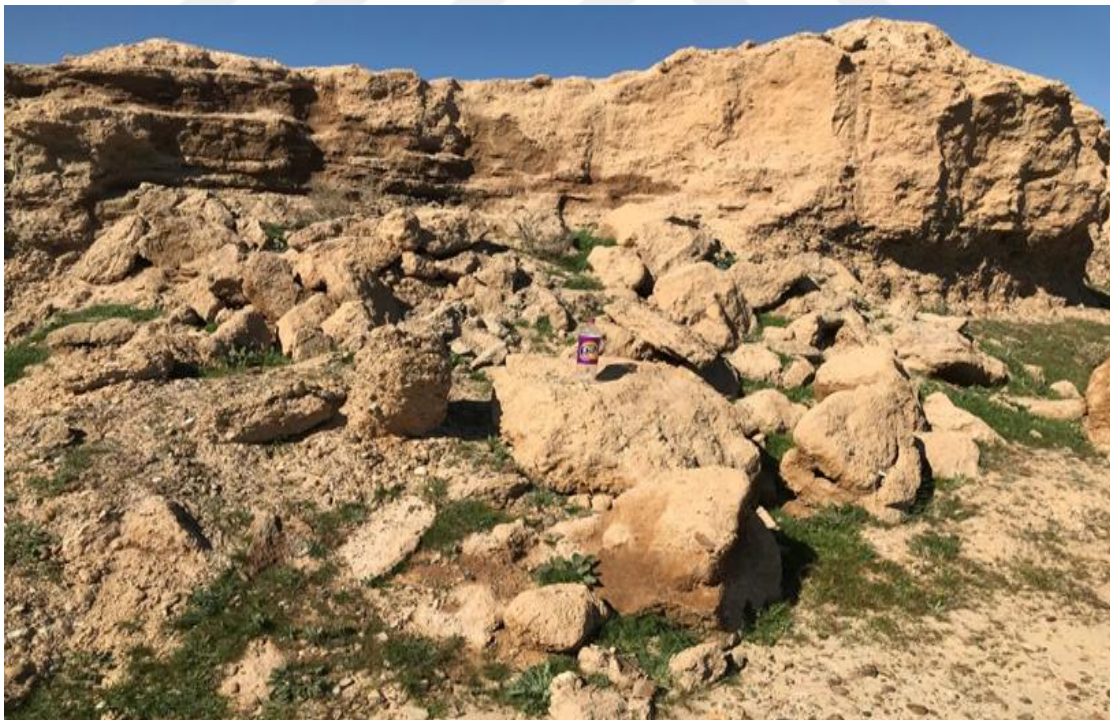
Photograph 18. Rockfall near the Al-Samtheai Village
