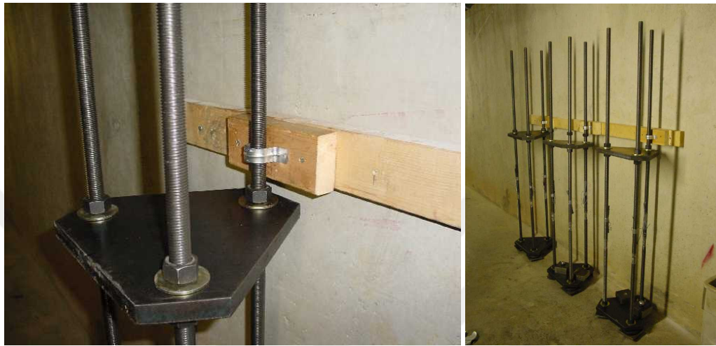
Figure 3-26 – Erection of the Creep Rack
