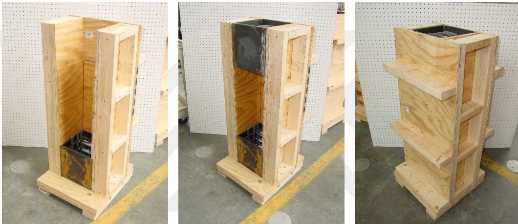
Figure 3-9 – Assembly of the Formwork
