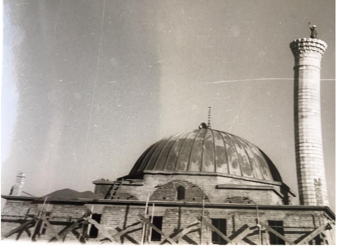
Figure 3. 20. Erenköy Mosque Under Construction, 1971 (Büyükkörükçü Archive)
