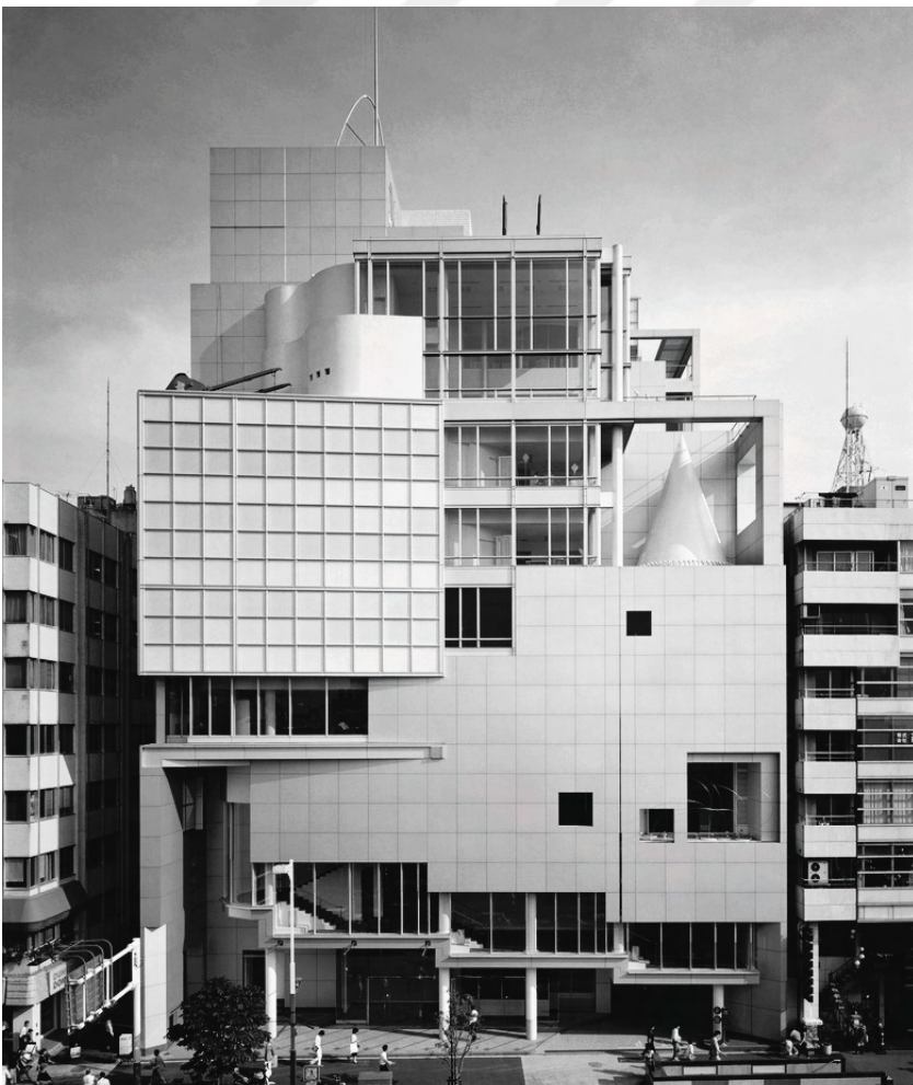
10 The Spiral by Fumihiko Maki (completed in 1985)
