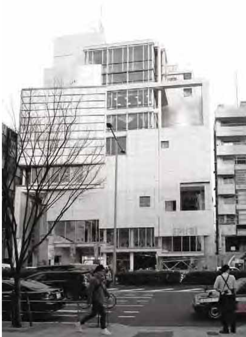
24 Spiral exterior view (right) and the spiral ramp in the building (opposite)
