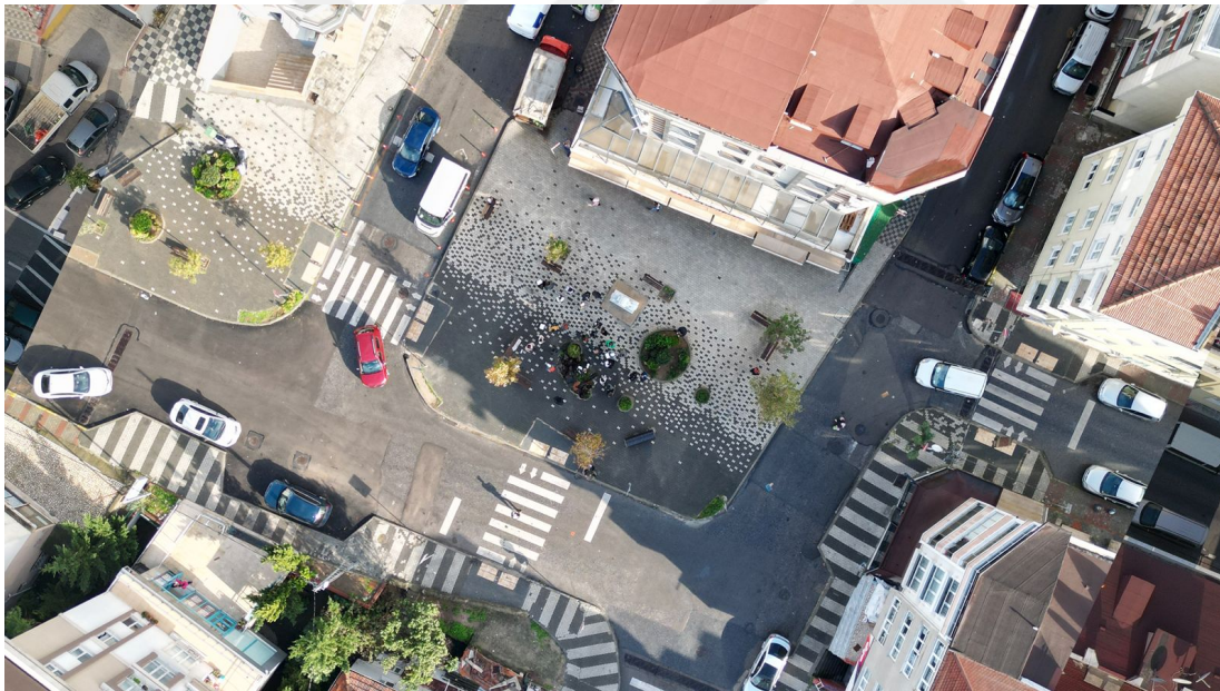
Figure 3.18 : The drone view of the area after permanent street transformation (Superpool, 2020)
