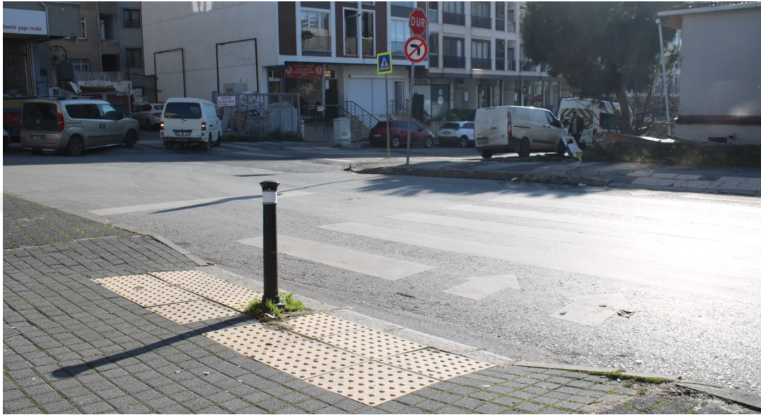
Figure 4.11 : A bollard on the disabled ramp and in front of the pedestrian crossing
