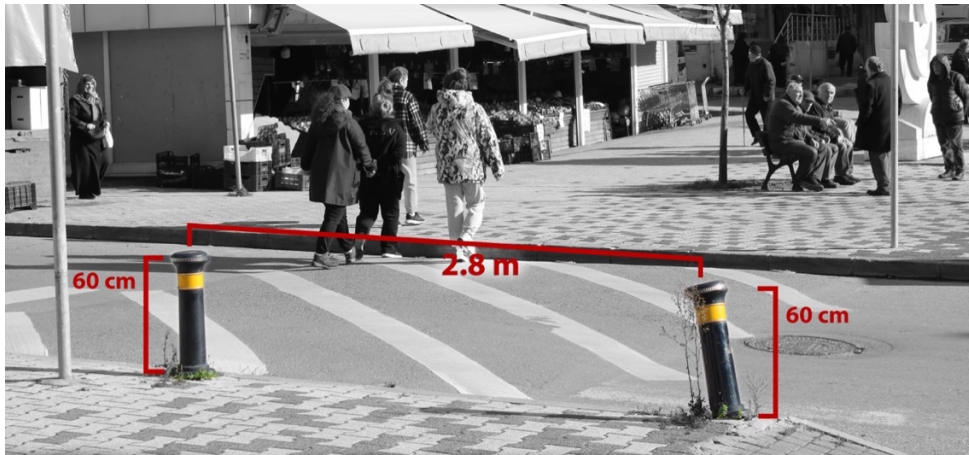
Figure 4.30 : Distance between bollards and their measurements
