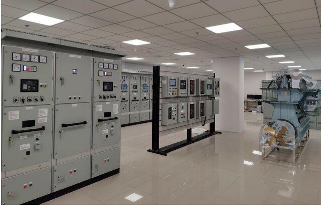
Őekil 2. Makine Dairesi Simlatr
