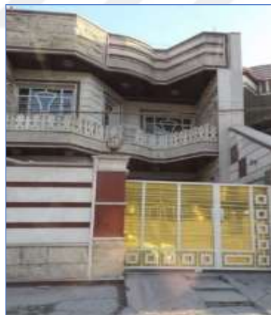
Figure 2.29: Photos Show the Façade of Zahraa ALBUNDI'S House in Baghdad.
