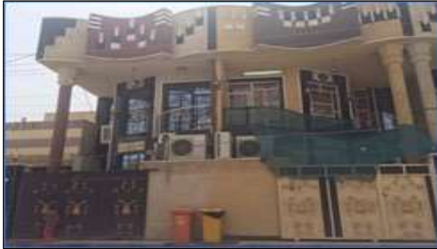
Figure 2.38: The Facades of QAIS ALMAAMORYS House.
