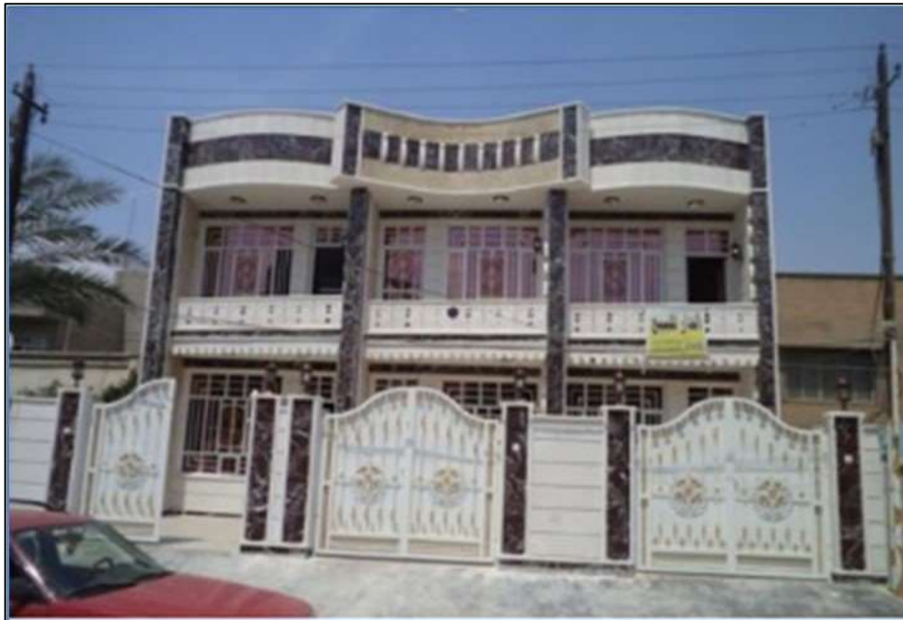
Figure 2.40: The Facade of ABDUL ALRASHEEDYS House.
