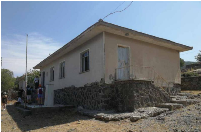
Figure 3.2. Yahşibey new school building before adaptive reuse proposal (Yahşibey Tasarım Çalışmaları, 2022).
