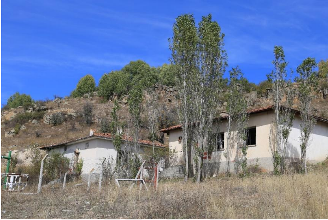
Figure 5.24. Berçinçatak Village abandoned school.
