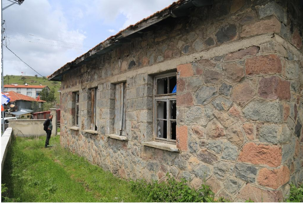
Figure 5.37. Süleler Village abandoned school.
