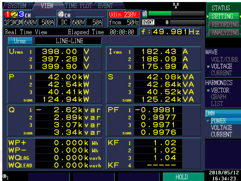
Figure 4-41 Line-to-line voltages, line currents, power drawn from the grid, and power factor
