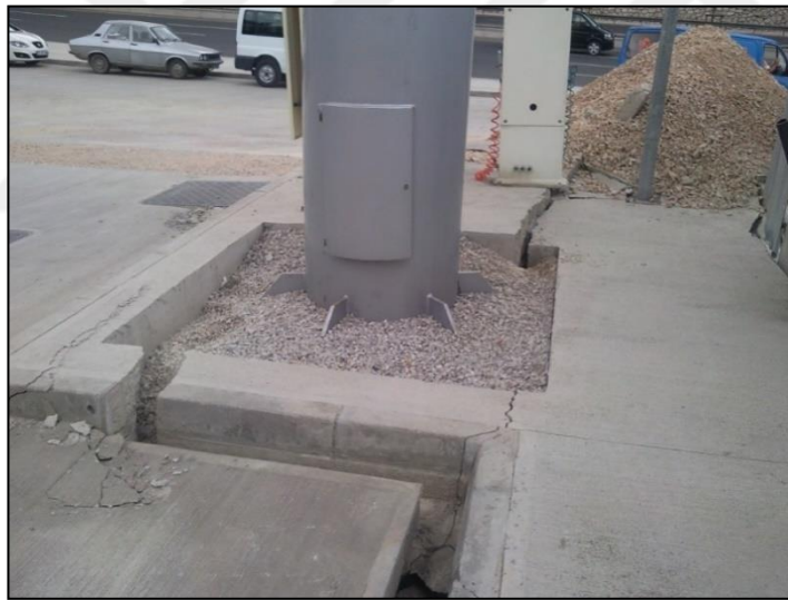
Figure 4.9. Crack formations observed in the gas station due to the ground deformations caused by the foundation excavation (Bakır, 2011).
