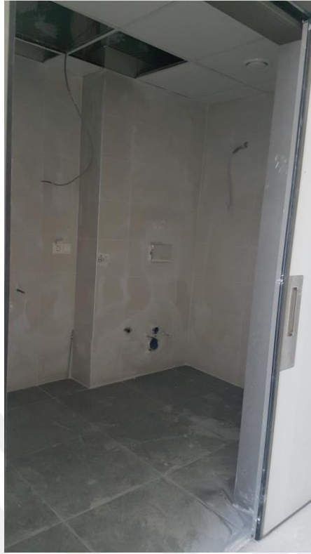
Figure 0.3. E. Picture#3 of Hospital Private Room #1
