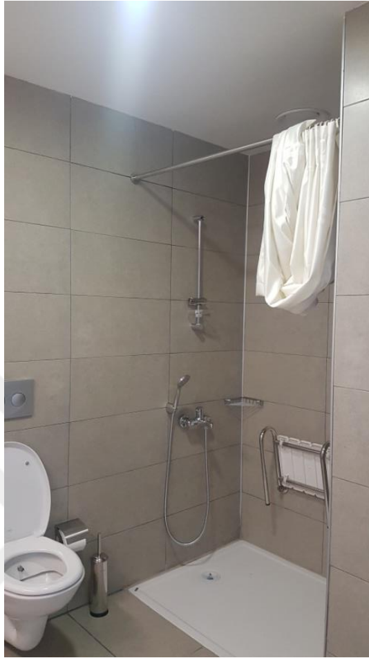
Figure 0.15. E. Picture#3 of Hospital Private Room #4
