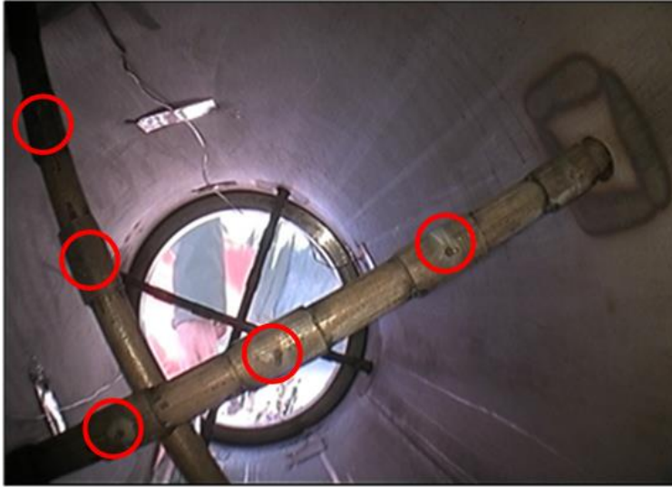
Figure 4.22: Temperature measurement rakes inside the CAH.
