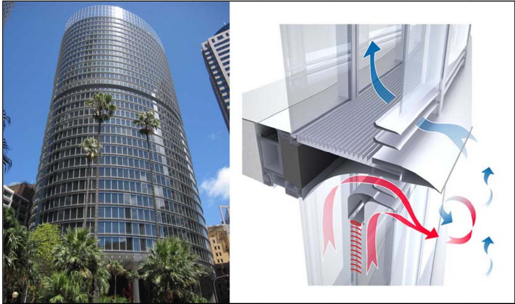
Figure 2.16. 1 Blight Street Tower-general view and aerofoil shaped louvers (courtesy of Ingenhoven Architects)
