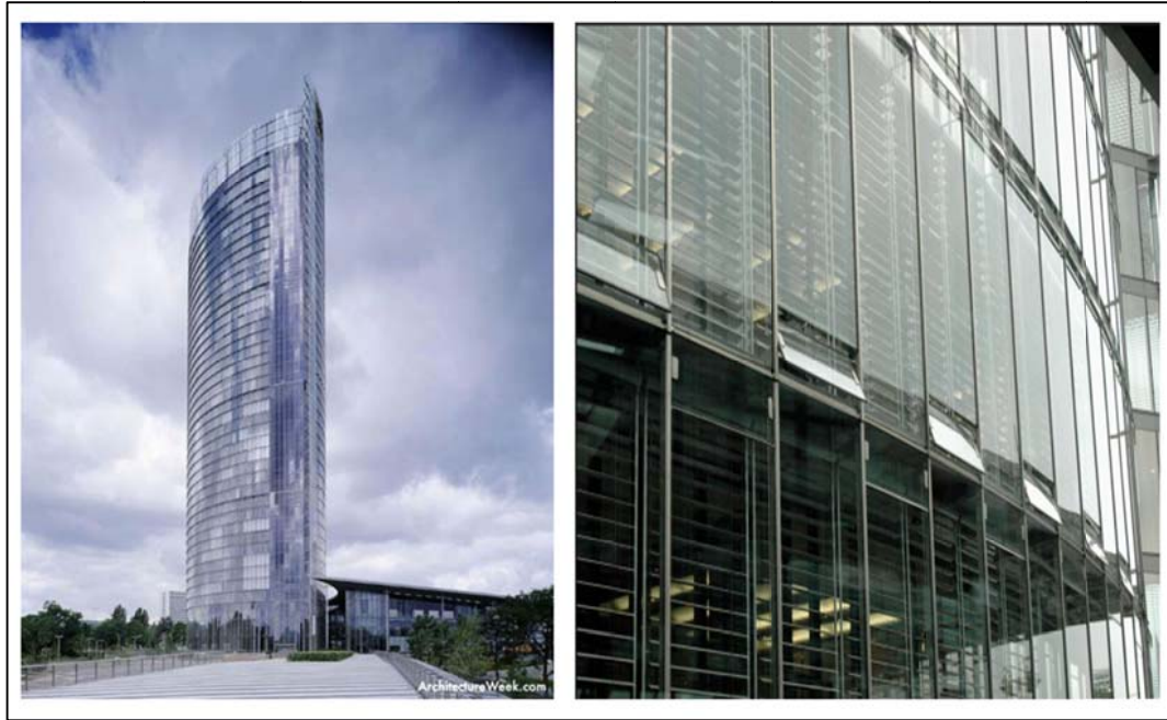
Figure 2.14. Post Tower- general view and highly reflective, adjustable blinds (courtesy of Murphy/Jahn Architects)
