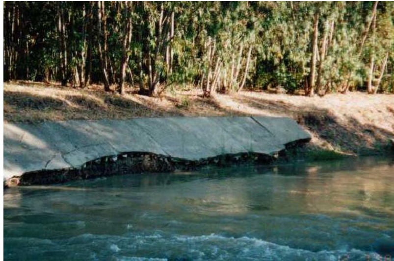
Figure 5.8. Collapsed river bank located on the failed embankment (Japan Society of Civil Engineering Reports, 1998).
