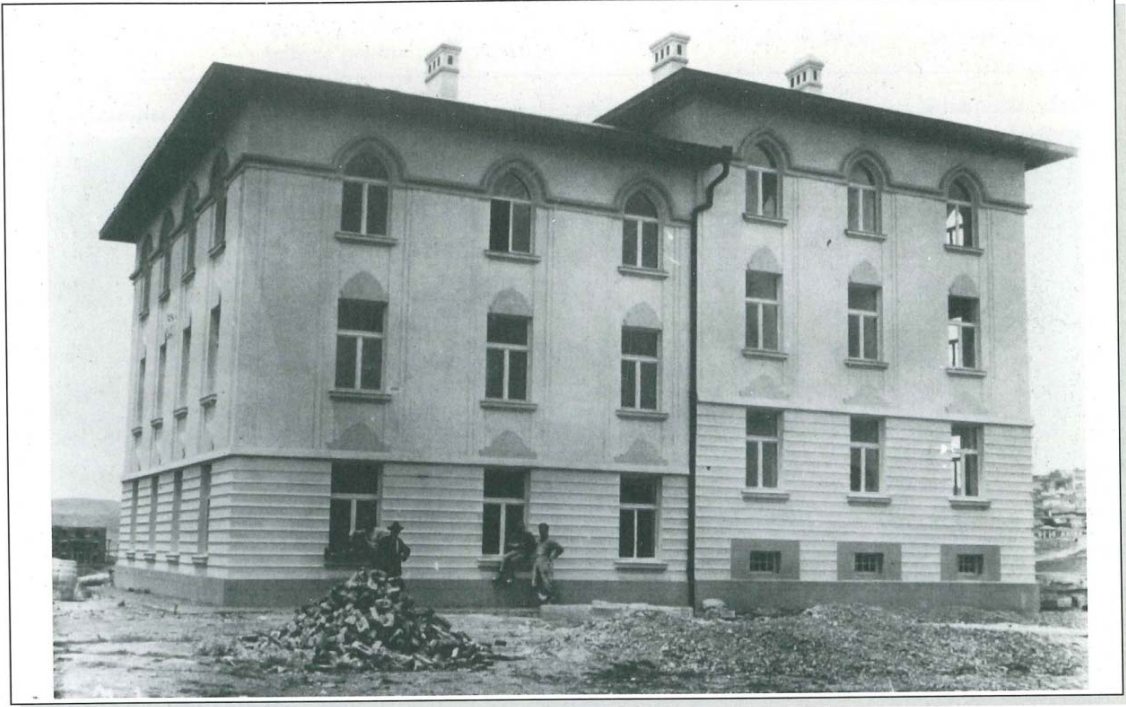
Yenisehir'de bir inşaat (1928-29) A Construction of a building in Yenisehir (New City)
