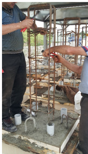
Figure 2.6: Reinforcement of cages: (a) Stub cage. (b) Stub cage with column longitudinal bars. (c) Plan view of stub cage. (d) Stirrup with 90° hook angle. (e) Assembling of stirrups. (f) Plan view of column cages
