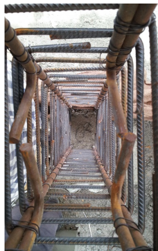
Figure 2.6: Reinforcement of cages: (a) Stub cage. (b) Stub cage with column longitudinal bars. (c) Plan view of stub cage. (d) Stirrup with 90° hook angle. (e) Assembling of stirrups. (f) Plan view of column cages
