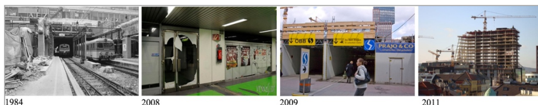
Figure 1.5 : Wien Mitte Station Refurbishment Process (Url-1).
