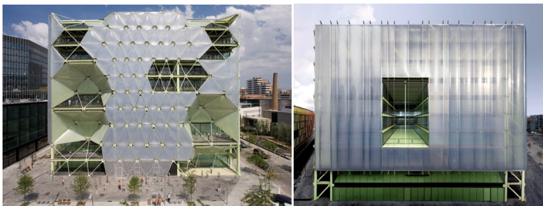
Figure 2.5 : Media-ICT Façade, Cloud 9, 2010 (Url-7).
