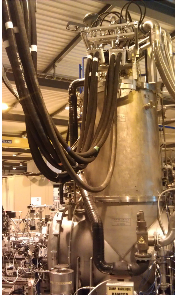
Figure 4.4. Magnet feed box and flexible lines.
