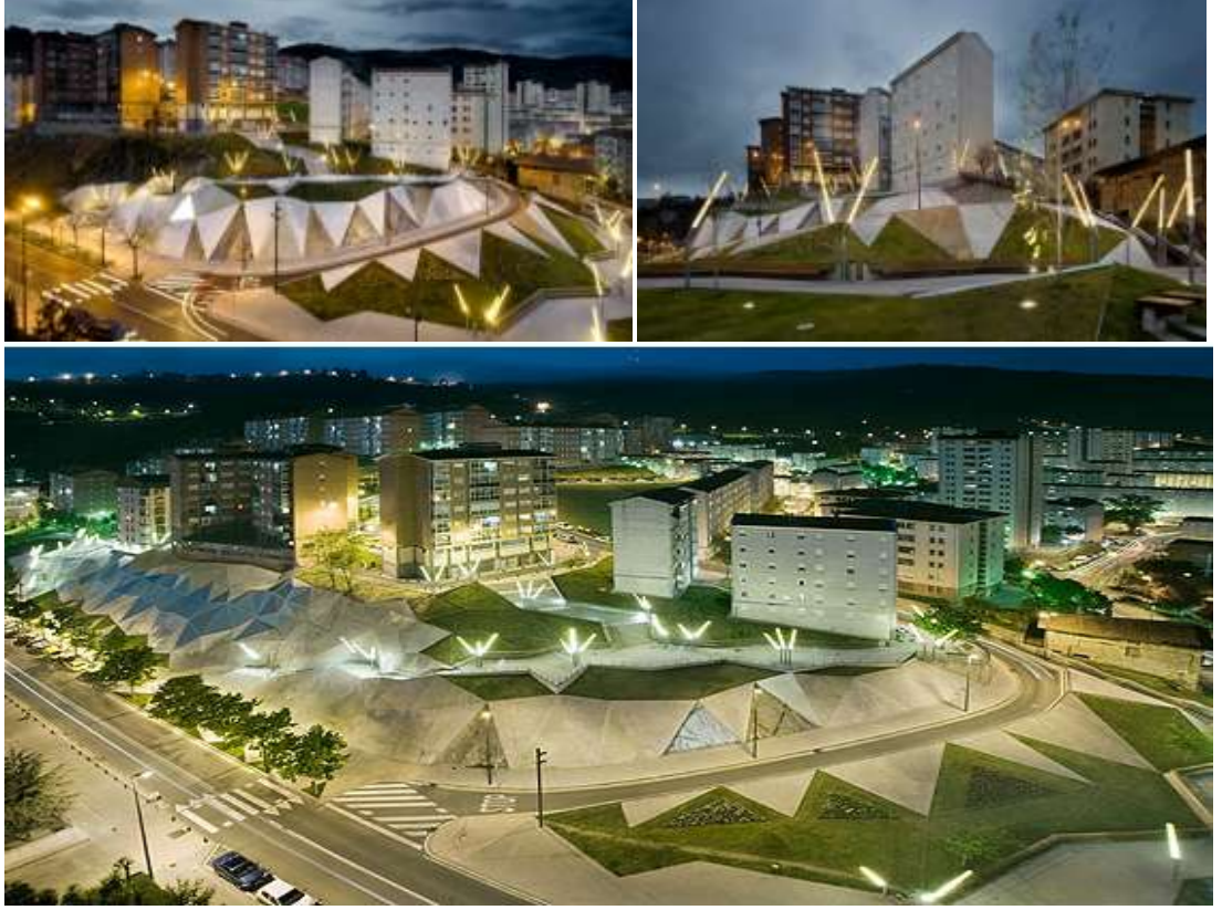
Şekil 3.18. Galindez Slope And Pau Casals Square
