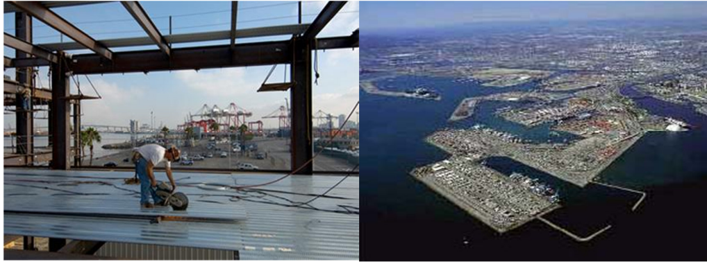
Figure 4.10 Long Beach Building New Piers
