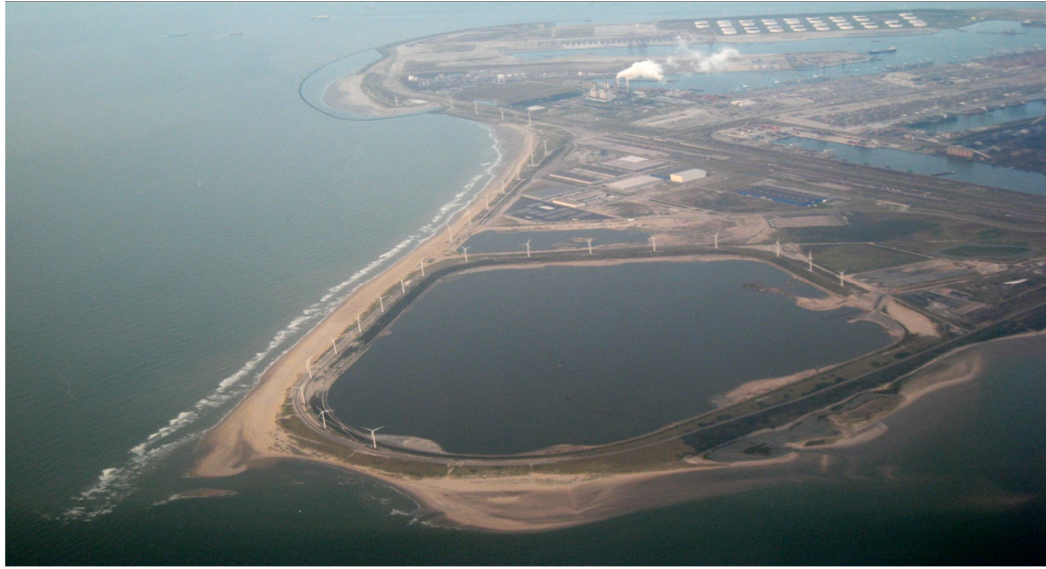
Figure 4.9 Maasvlakte-additional part of Rotterdam port
