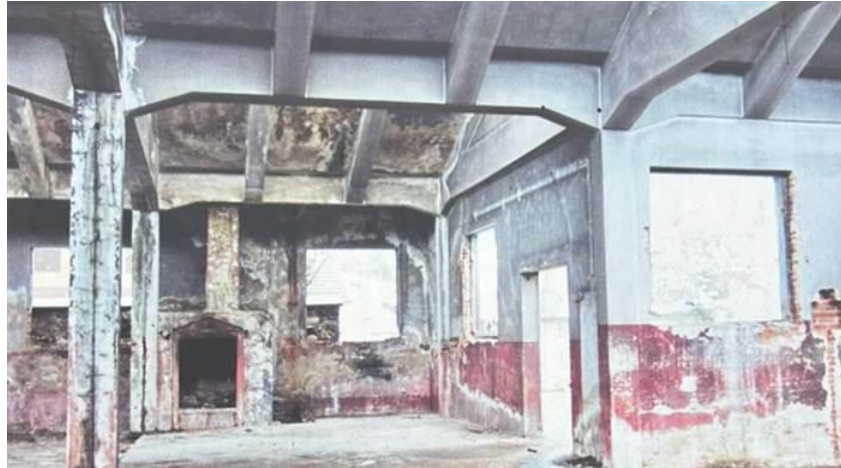
Figure 61. The structure of the building (Naim Arnas Archives, 1998).
