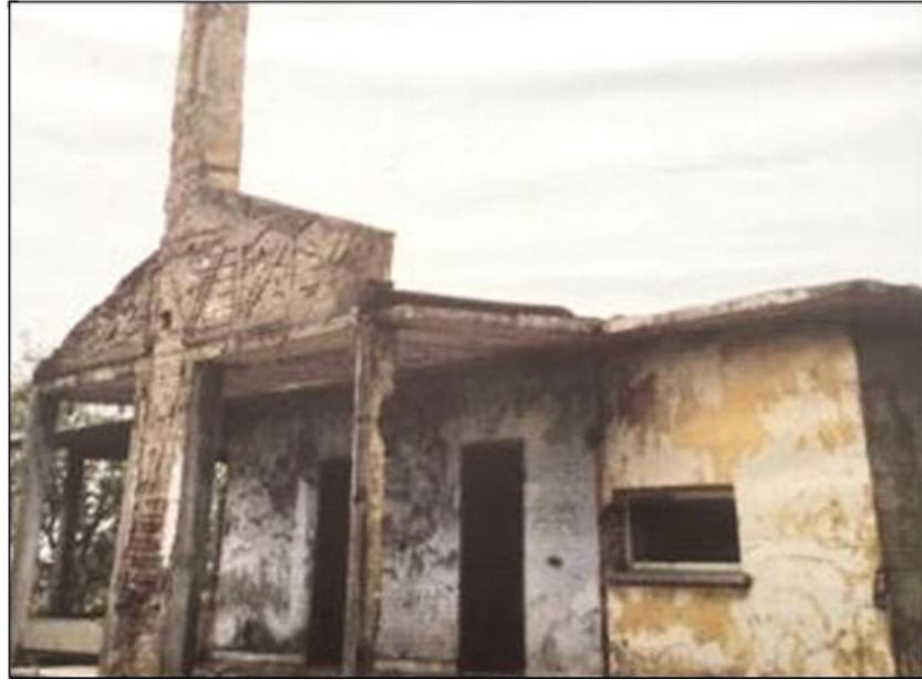
Figure 94. An image of the outbuilding before the restoration (Doğanlar, 2018).
