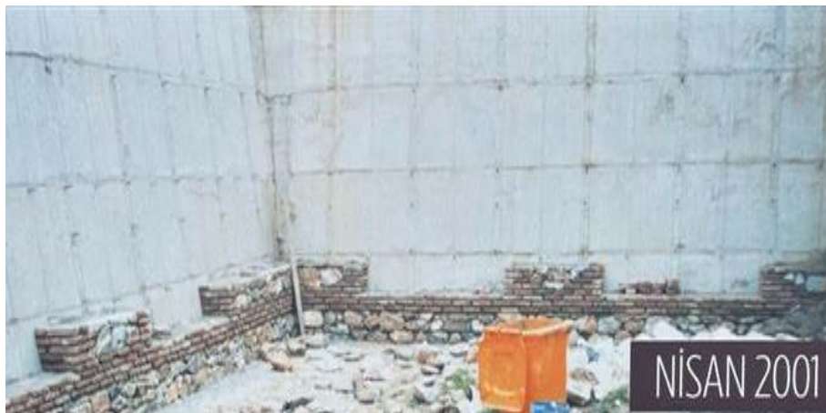
Figure 44. Strengthening works in Mancınikhane in the Ipeker factory in 2001 (Naim Arnas Archives, 2000).
