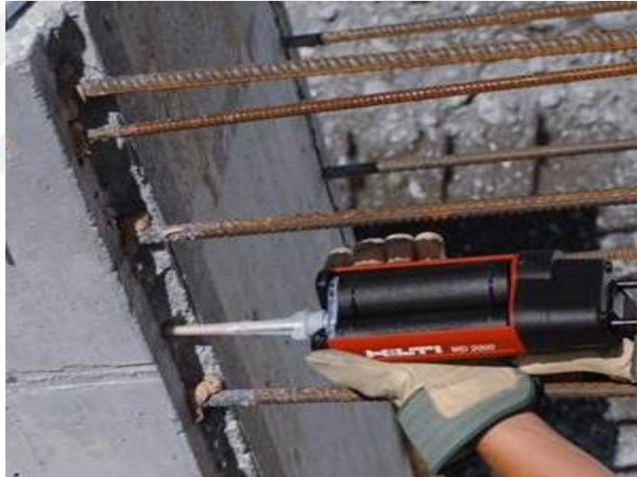
Figure 59. Filling the holes on concrete with epoxy dowels using the “Hilti” machine (hilti.com.tr, 2024).
