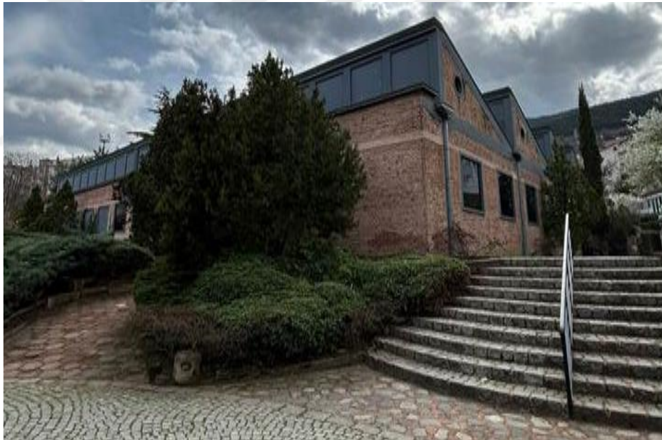
Figure 48. The museum's façade taken from the lower grade (Author's Archive, 2023).
