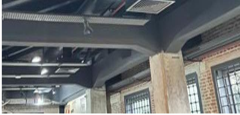
Figure 62. An image of the beams that are painted black (Author's Archive, 2024).
