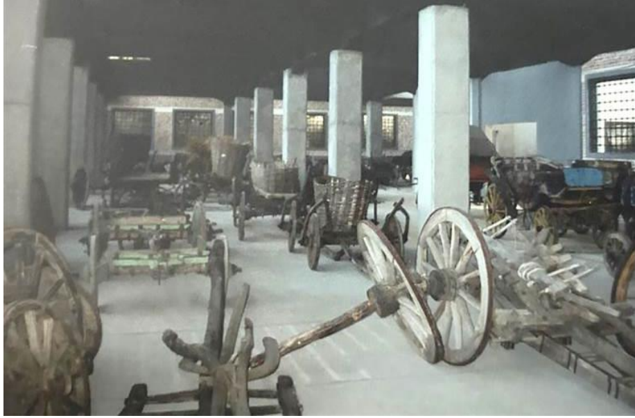
Figure 66. Strengthened 60 x 60 columns and some of the carriages from the exhibition's first section (Mehmet Batıtürk Archives, 2001).
