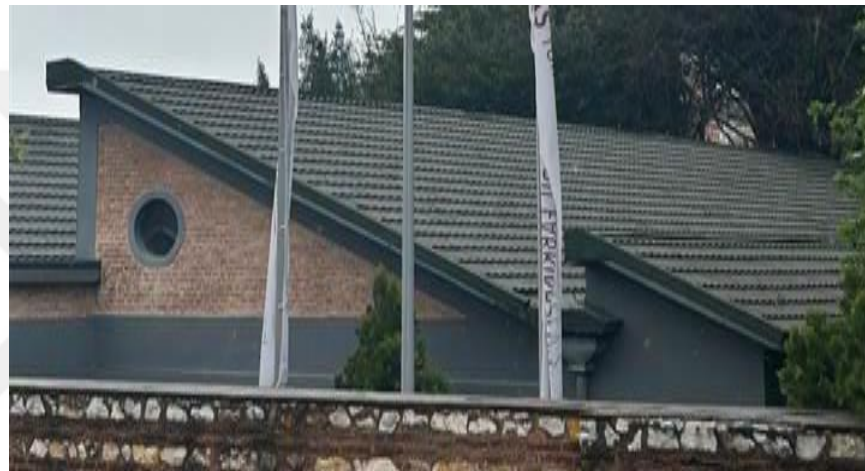
Figure 81. An image of the roof and circular window (Author's Archive, 2024).
