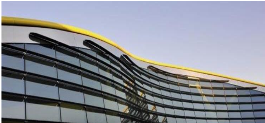
Figure 6. The curtain wall façade that faces towards the Enzo Ferrari's house (ArchDaily,2012).
