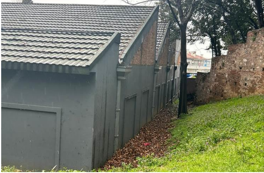
Figure 68. The back façade of the building where the window openings are closed and east and south facades painted with smoky grey paint (Author's Archive, 2024).
