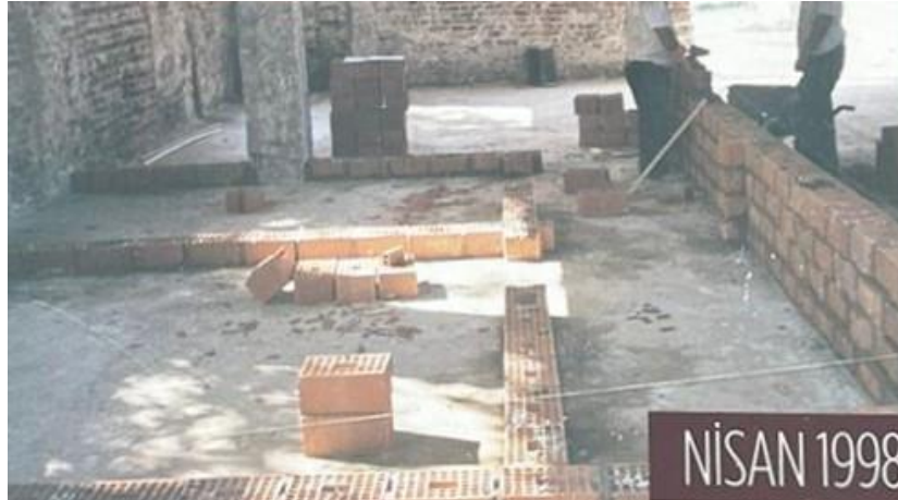
Figure 83. The building of the 20 cm interior brick walls in 1998 (Author's Archive, 1998).
