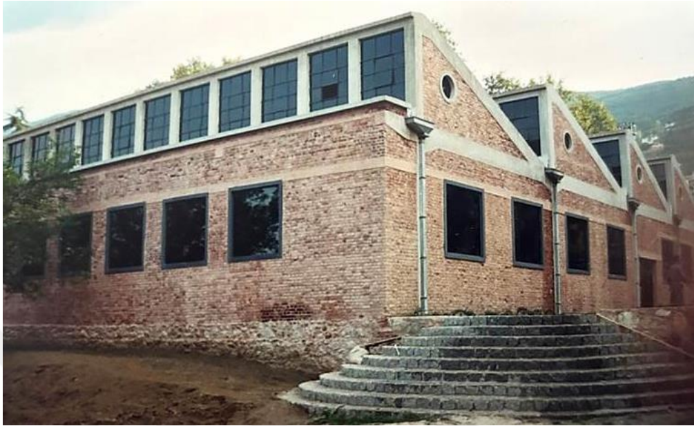
Figure 72. The exterior brick walls and windows after their renovation (Mehmet Batıtürk Archives, 1999).
