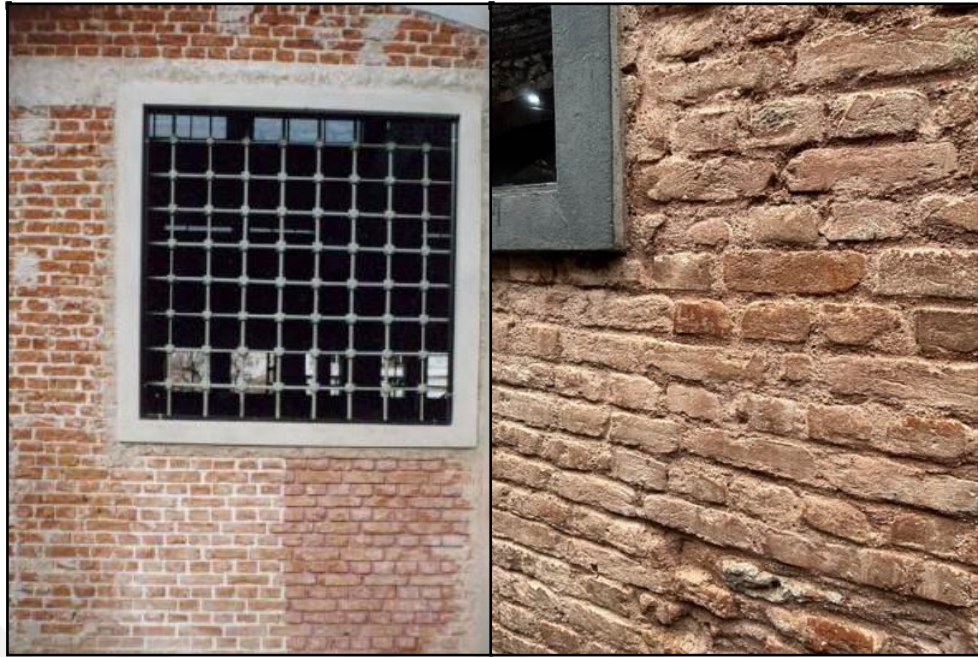
Figure 70. The exterior brick walls in 1998 on the left and applied red mortar joints on the right (Naim Arnas Archives, 1998&2024).
