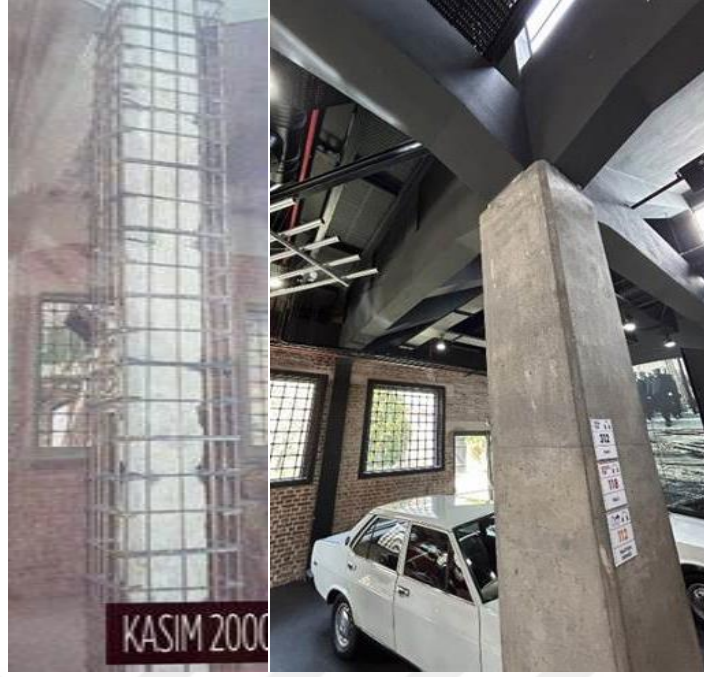
Figure 58. The strengthening operations on the columns on the left and 60 cm x 60 cm column on the right (Author's Archive, 2024)
