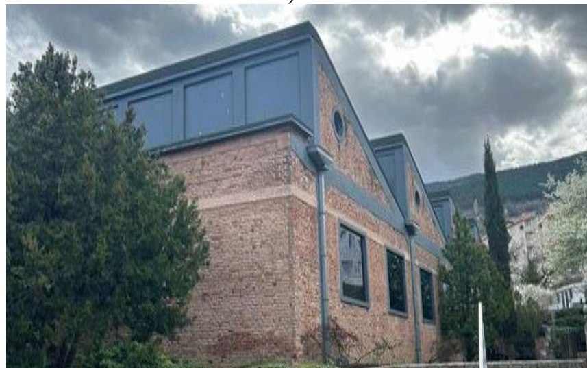
Figure 82. The square windows that are cancelled and painted with smoky grey paint (Author's Archive, 2024).
