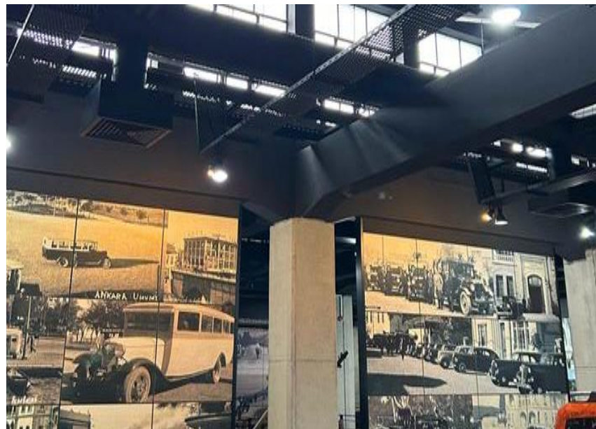
Figure 75. The beams covered with black paint (Author's Archive, 2024).
