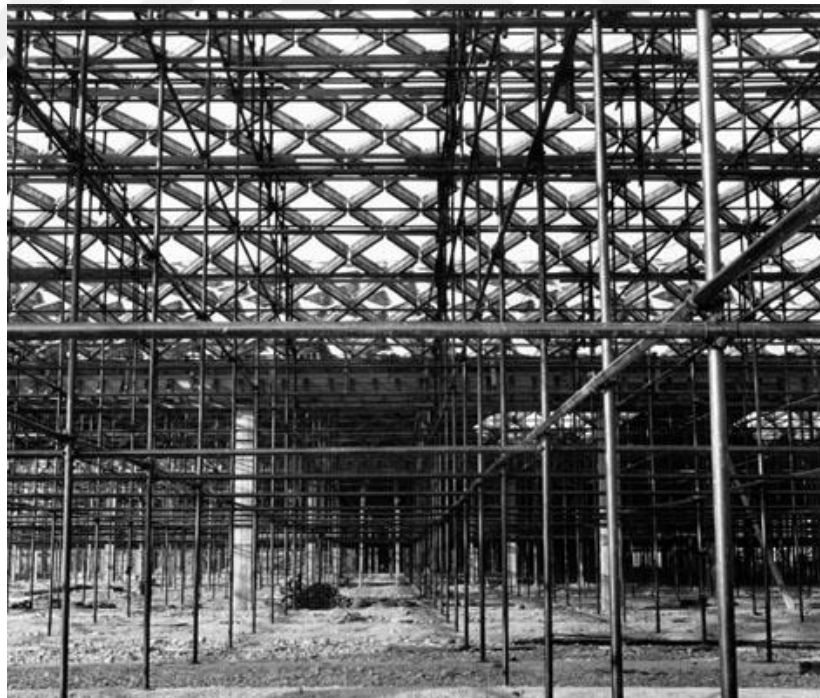
Figure 32. Construction of the plant in Arese in 1966 ( museoalfaromeo.com , 2016).
