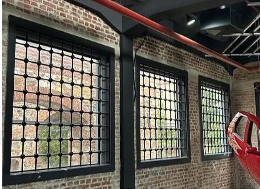
Figure 74. The iron ball-tipped railings on the interior (Author's Archive, 2024).
