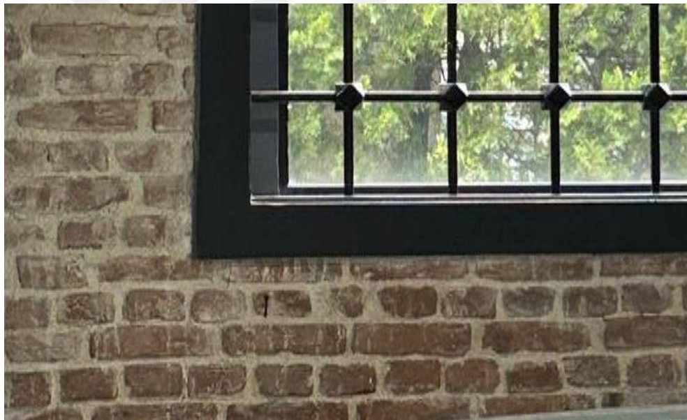
Figure 71. Brick walls with white mortar joints applied on the interior (Author's Archive, 2024).
