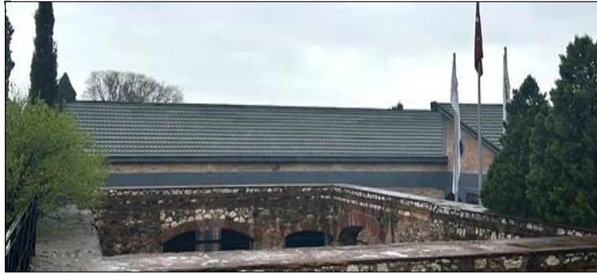
Figure 80. An image of the roof (Author's Archive, 2024).
