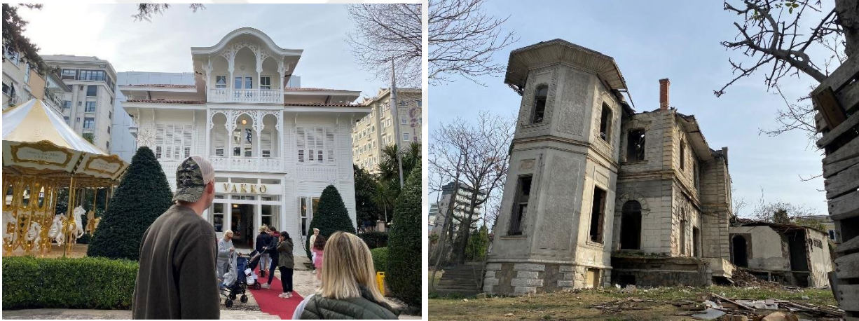
Image 36 On the left is the Mehmet Küçükdeveci Bey Mansion, currently used as the Suadiye Vakko store, and on the right is the Tamara Mansion, which is on the verge of collapse. Photos by the author.
