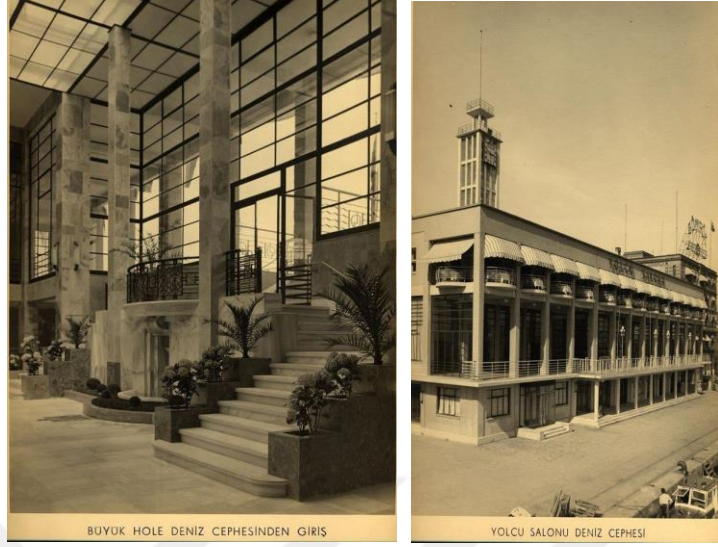
Figure 13. (Karaköy Passenger hall during pas times from interior and exterior perspective)
