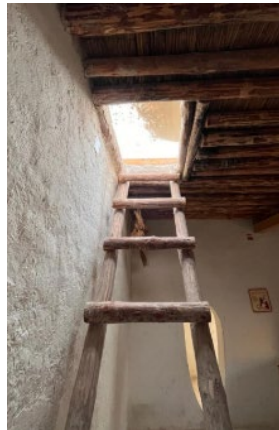
Figure 10. Entrance to the house with wooden stairs from the roof (Author, 2022).
