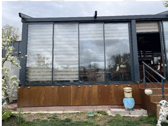
Figure 116. Storage spaces under the tiny house of resident B.3 (Author, 2024).
