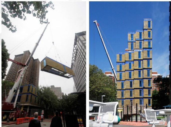
Figure 34. Prefabricated units of Carmel Place (Kolson Hurley & Volner, 2017).
