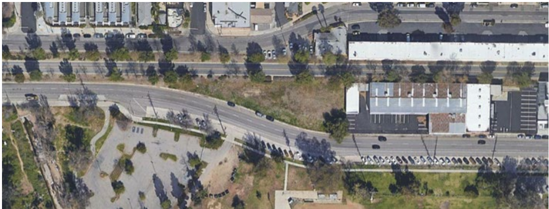
Figure 56. Site of the Chandler boulevard bridge house village before construction (Craft, 2021).
