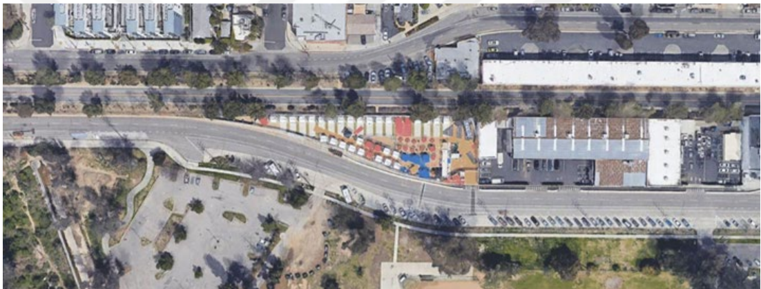
Figure 57. Site of the Chandler boulevard bridge house village after construction (Craft, 2021).
