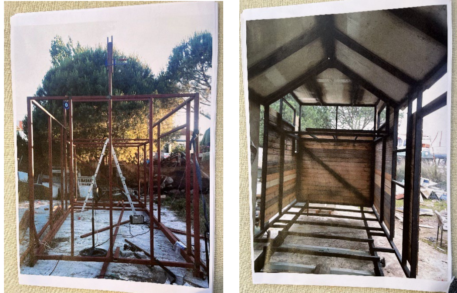
Figure 112. Photographs illustrating the construction process of the tiny house, as shown by resident A.2 (Author, 2024).
