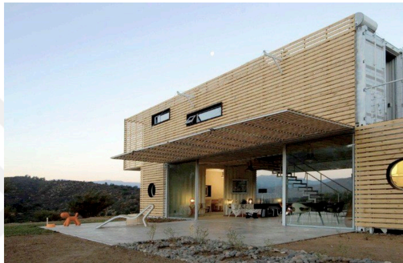
Figure 42. The Manifesto shipping container house (Derringer, 2010).
