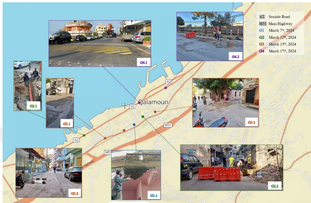
Figure 15. Map and photographs of observed structure work in Qalamoun, by author
