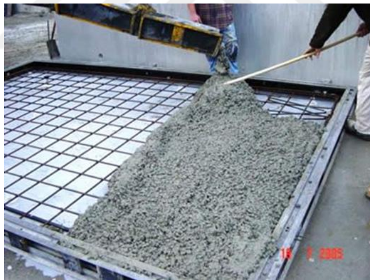
Figure 15. Casting of EPS mold. (Lcf center)
