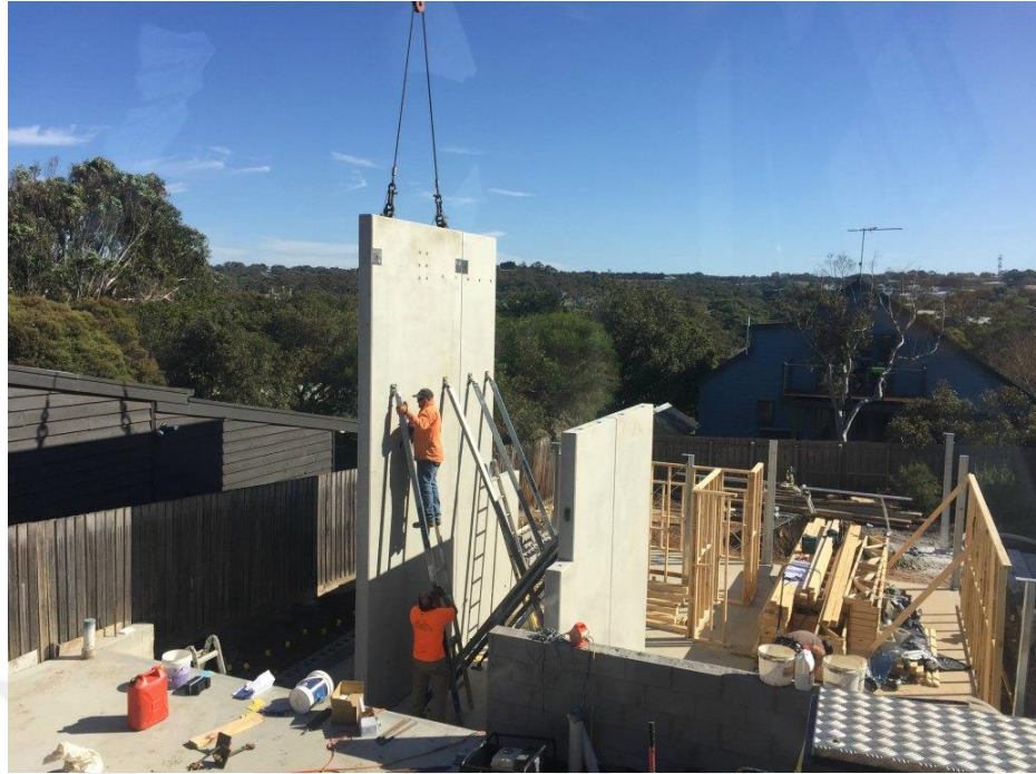
Figure 14. Precast construction. (Otway precast)
