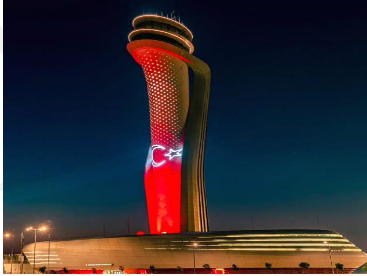
Figure 13 Istanbul Airport's Tulip-Shaped Control Tower 12
