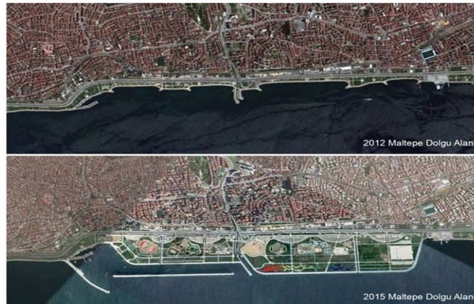
Figure 2.14: Satellite image of the filled sea (Url-14).
