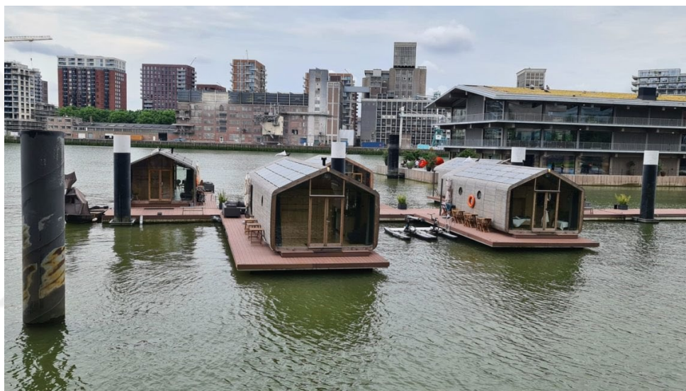
Figure 2.2: Floating office (Url-2).
