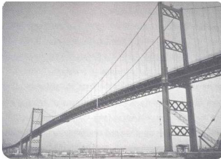
Figure 3.16. Photograph of the Vincent Thomas Bridge (Pridham and Wilson, 2002)
