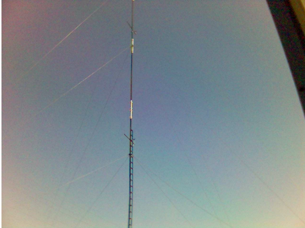
Figure 3.3 The erected mast.
