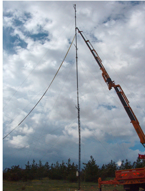
Figure AC.2 Erection of Mast (part 2)
