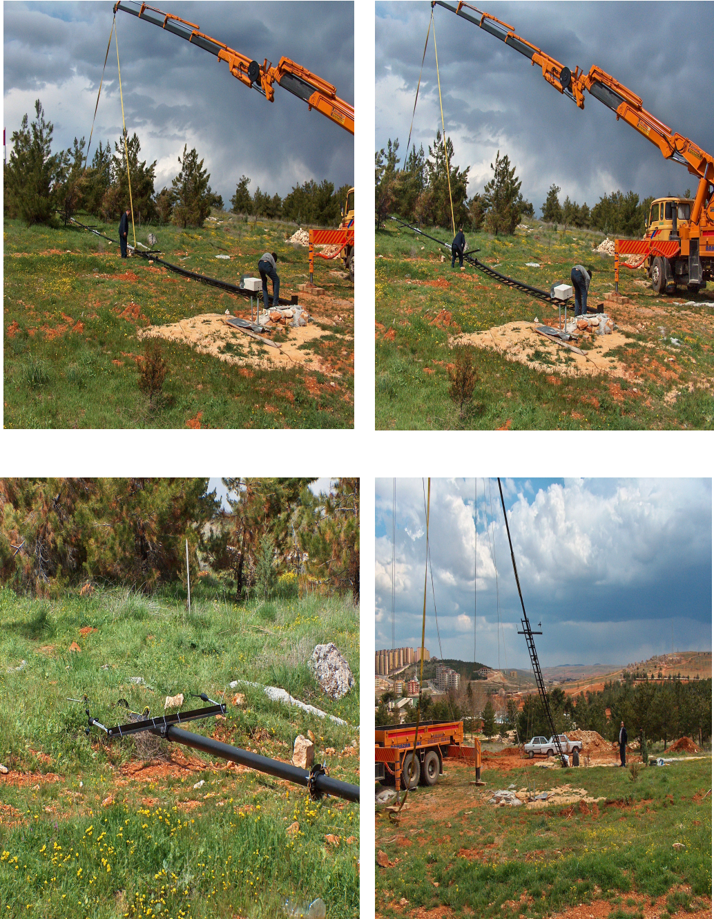
Figure AC.1 Erection of Mast (part 1)
