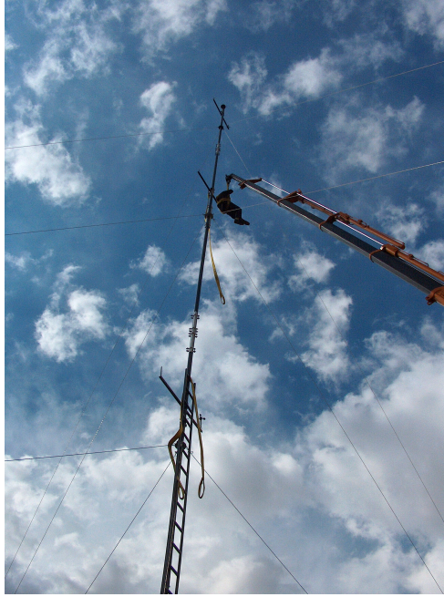
Figure AC.3 Erection of Mast (part 3)
