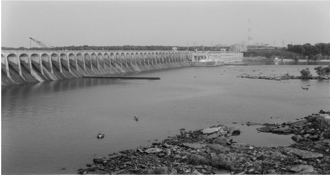
Figure 2.5. A buttress dam in the USA.
