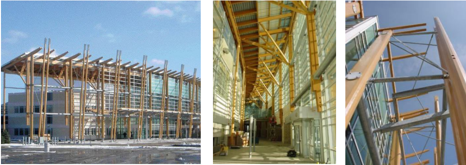
Şekil 3.27 – 3.28 – 3.29 : Regional Hospital, Thunder Bay, Ontario, Canada[12]
