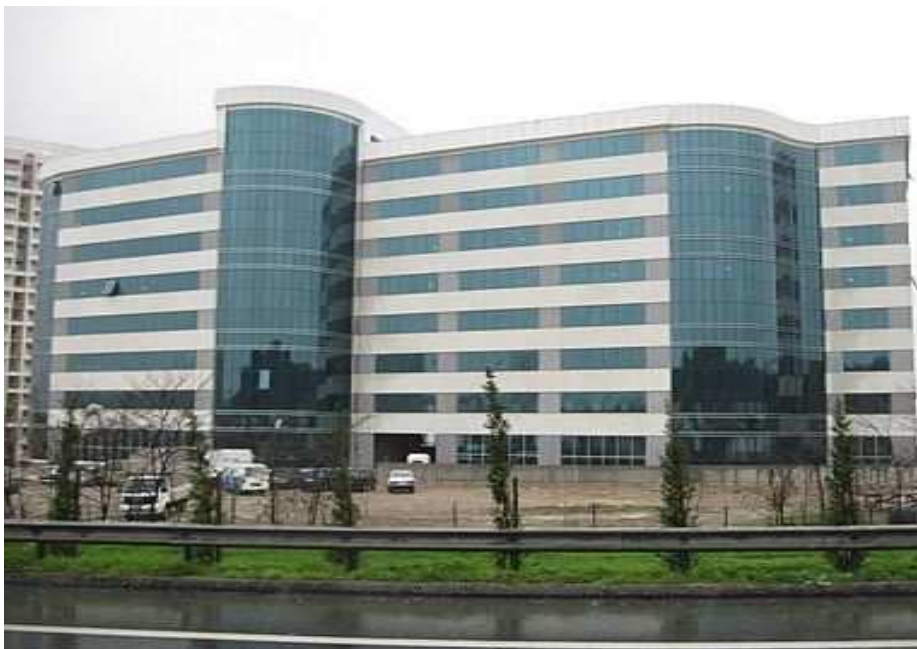
Figure 4.7 : Turkey's first LEED Certificated Office Building, Unilever Umraniye (source : Url-10)
