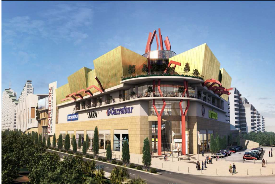
Figure 4.6: The Gordion Shopping Center in Turkey which has a BREEAM certificate. (source : Url-11)
