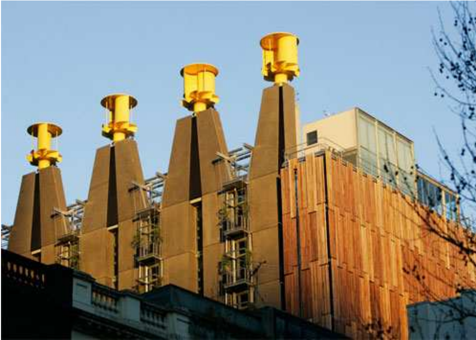
Figure 3.4 : Melbourne's Council House 2 in Australia. Wind turbines assist in the release of the building's exhaust (source: Url-6)
