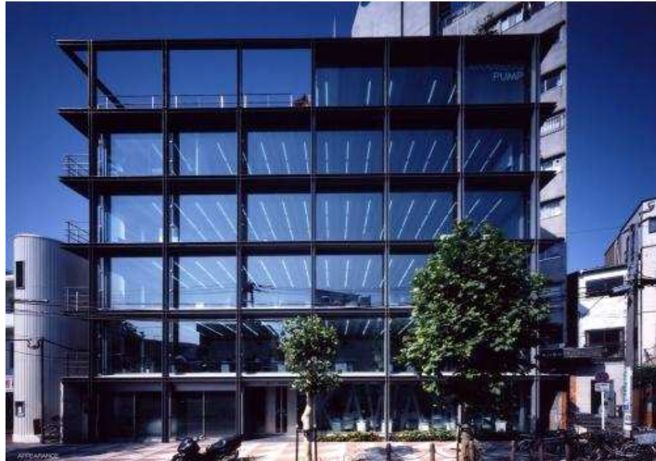
Figure 3.5 : Pump Manufacture Co Ltd, Tokyo Branch Building: Class A in CASBEE (source: Url-7)
