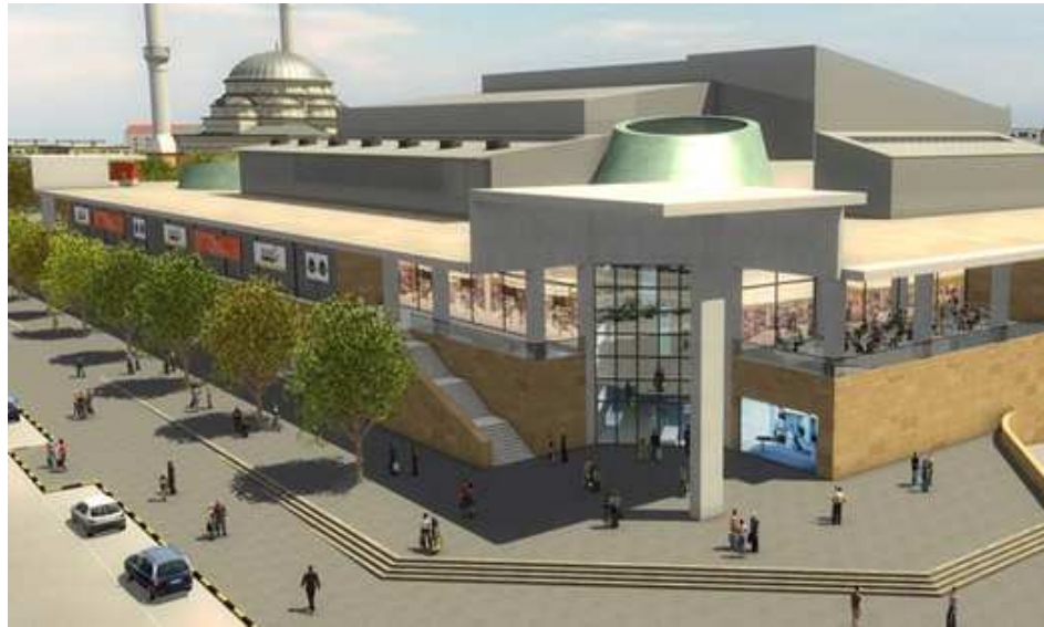
Figure 4.14 : Land View of Erzurum Shopping Centre
