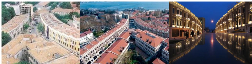
Figure 28: Akaretler – Before and after Renovation
