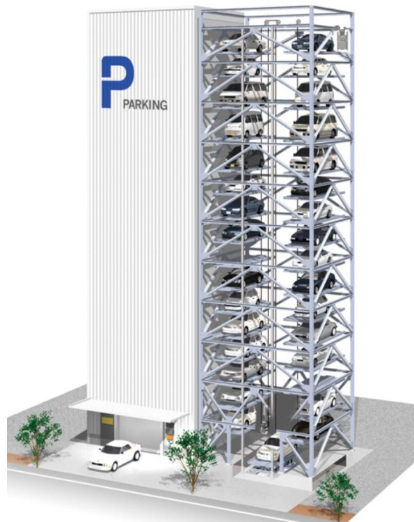
Figure 1.2 Modular tower-type AVPSS with an orientation of 2x1 (closed and open façade) (Web-japan, 2017)
