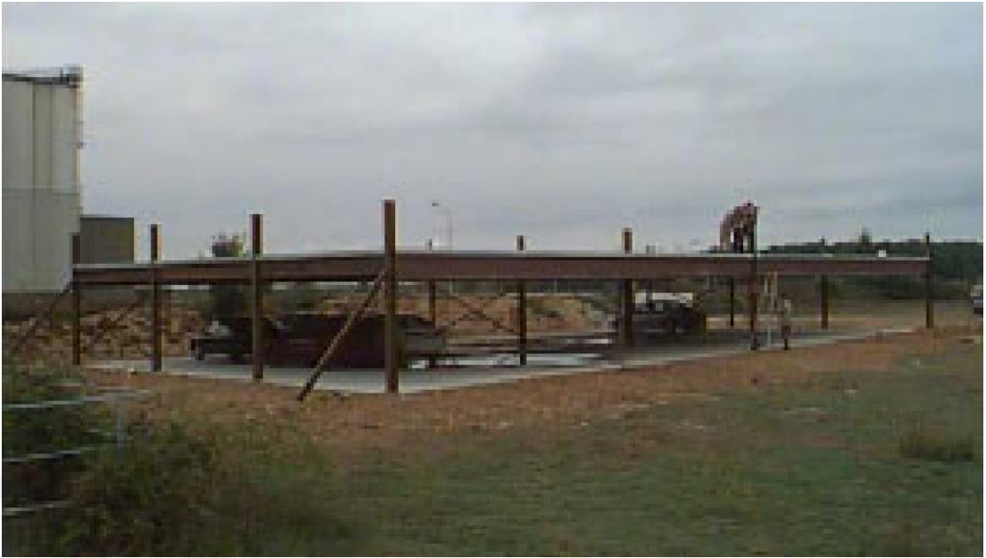
Figure 2.18 Open steel car park (Zhao and Kruppa, 2004)
