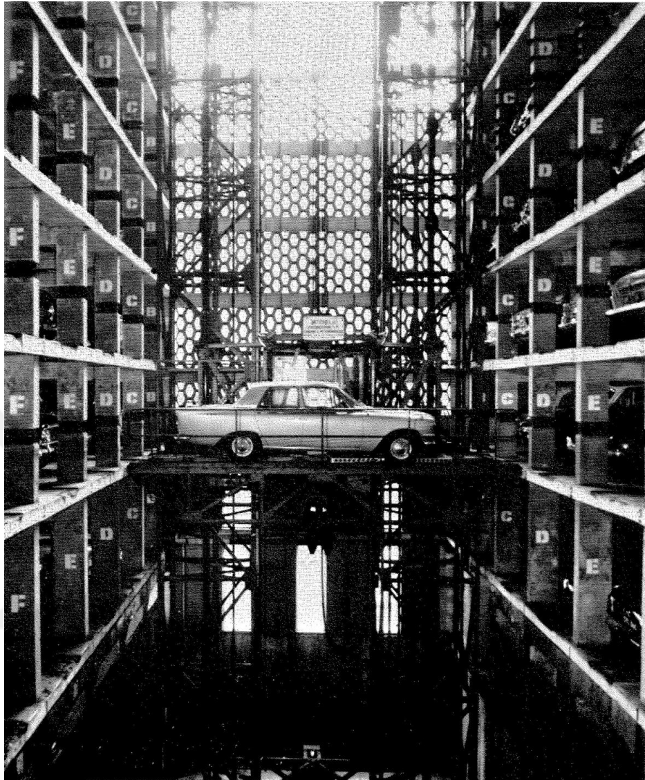
Figure 2.15 An early example of concrete AVPS in the 1970s (Dobson, 1974)
