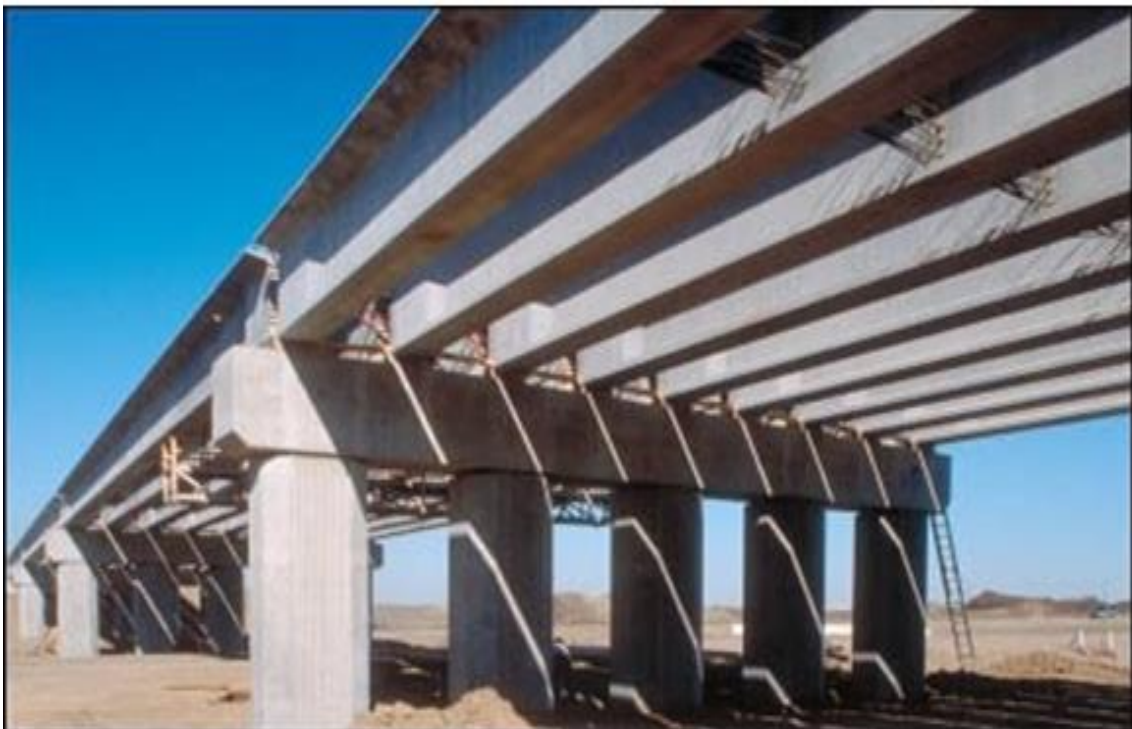
Figure1.1. An example of a bridge girder (Dana M Dietz 2017).
