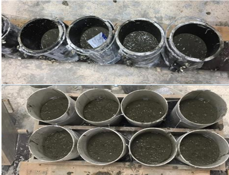
Figure 3.7. The first stage concreting.
