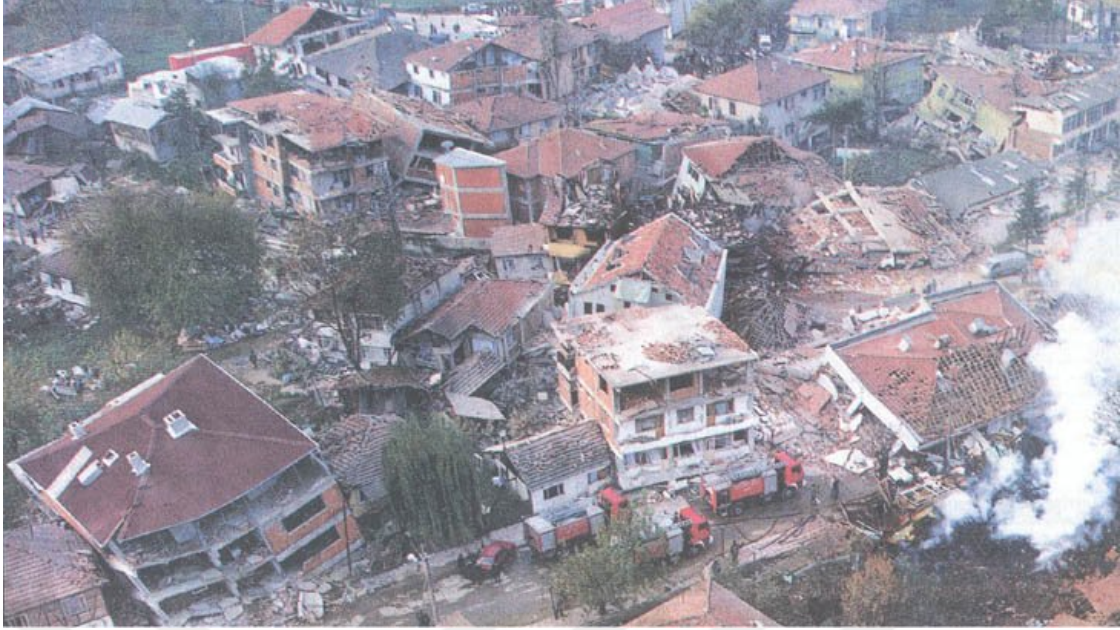
Figure 1.1 Damages and Collapses in Düzce City, www.koeri.boun.edu.tr
