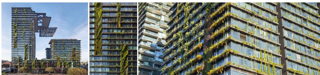
Figure 2.9: Building's carved deep vertical slots to allow light and air (Url-4).
