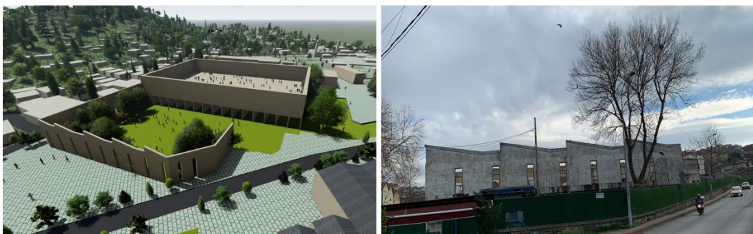
Figure 4.13: The industrial shed and the proposed proto-designed amphitheater (Left), following facadism (Right).
