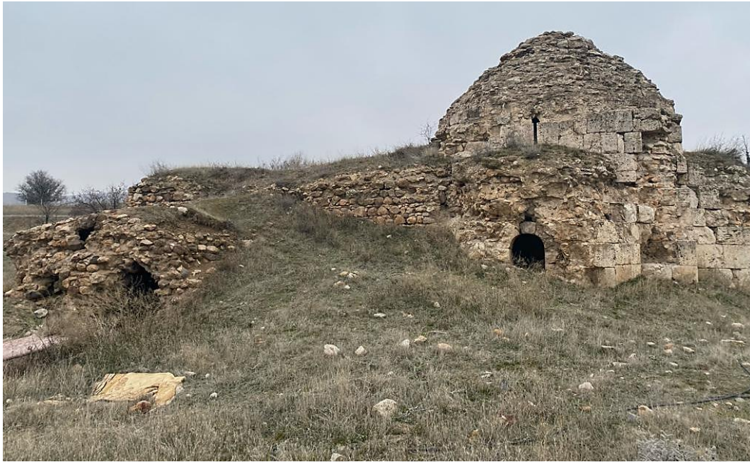
Figure 4.23. Burials observed in ground level in the area (Author's Archive, 2023)
