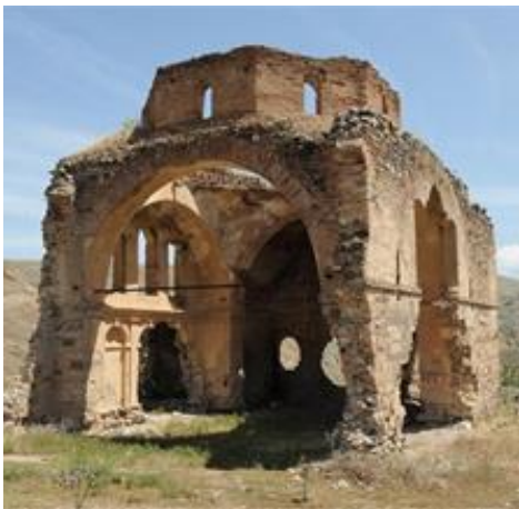
Figure 3.36. General View of Surp Lusavoriç Church (Source: https://tr.pinterest.com/pin/420242208969026242/ , Access Date: 05.11.2023)
