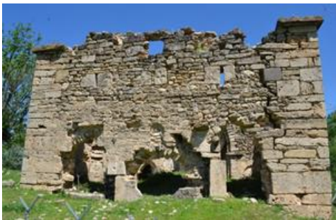
Figure 3.29. Ekinözü Church West Facade General View (Çapkur, 2023)
