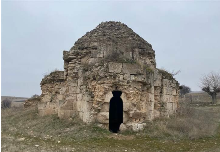
Figure 4.25. East Facade of the Church (Author's Archive, 2023)
