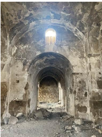
Figure 4.6. Transition from Naos Section to Jamatun (Source: Author's Archive, February 2023)
