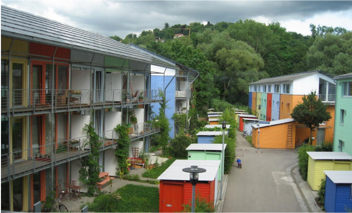
Figure 3.15. Freiburg is a Neighborhood with Solar Panels
