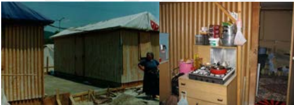
Figure 2.11 View of the two units and the concrete foundations for the kitchen in 2000 (left) and inside view of kitchen built between to the two paper houses in 2004 (right). (Johnson, 2008)
