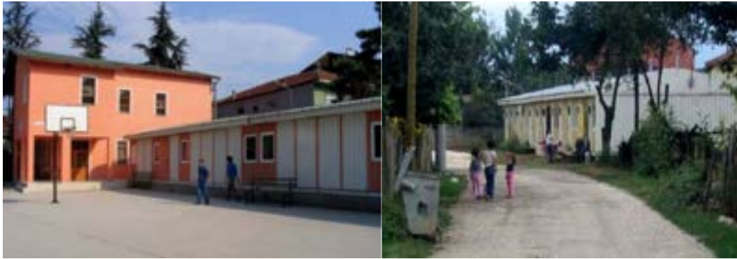
Figure 2.10 An eight-unit building that is part of the UMCOR temporary housing settlement (left); units reused as classrooms at a school (right) after being dismantled, moved across town and reassembled (Johnson, 2008).
