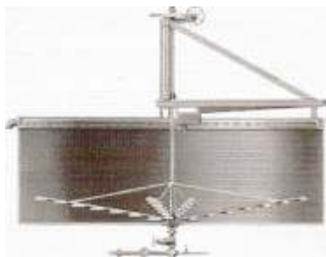
Figure 2.2 Original Dorr thickener (Dorr, 1936).
