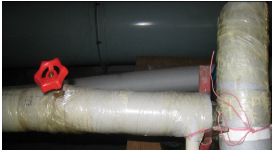
Figure 2.6 The flow adjustment valve
