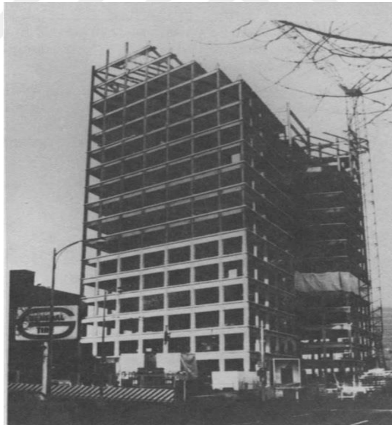
Figure 2.1 Moment-Resisting Frame (Popov, 1988)
