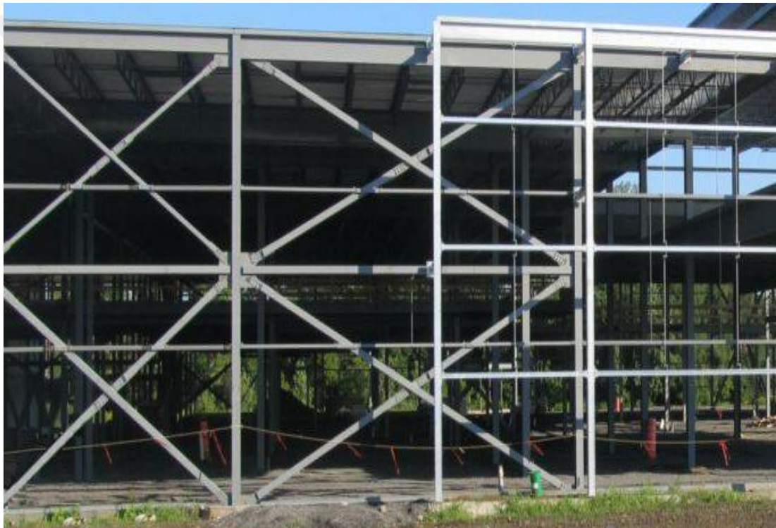
Figure 2.5 Steel Braced Frame
