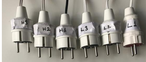
Figure 3.7. Plugs of the 6 lines of luminaires.
