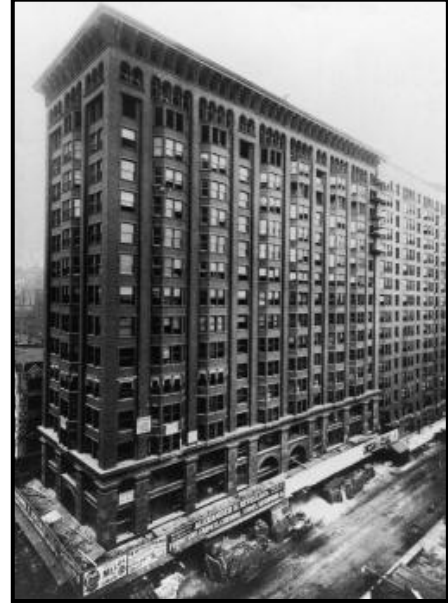
Resim 2.8. Monadnock Binası, Chicago 1893 ( http://www.monadnockbuilding.com/history.htm )
