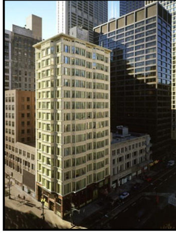
Resim 3.8. Reliance Binası ( http://www.arch.mcgill.ca/prof/sijpkcs/structures/reliance.jpg )
