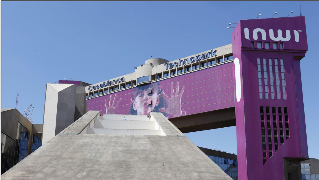
Figure 3.14: Technopark in the south of Casablanca built in 20
