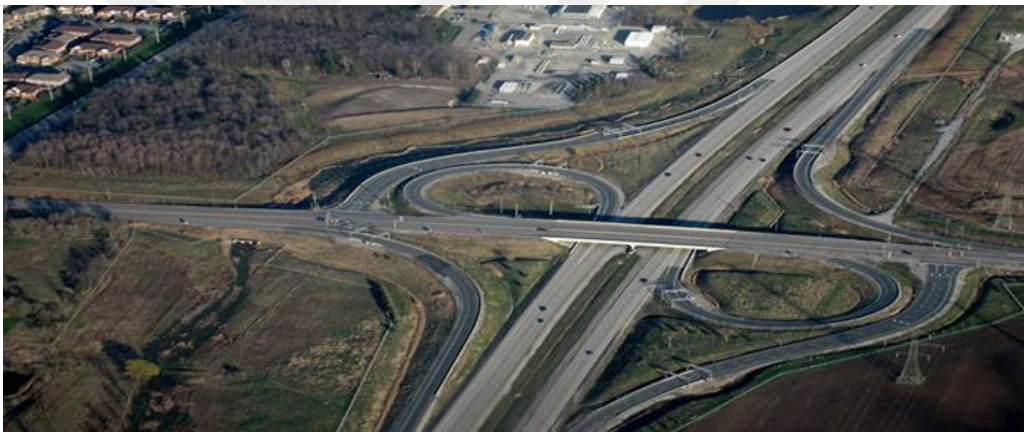
Figure 2. 20 Partial Cloverleaf Interchange
