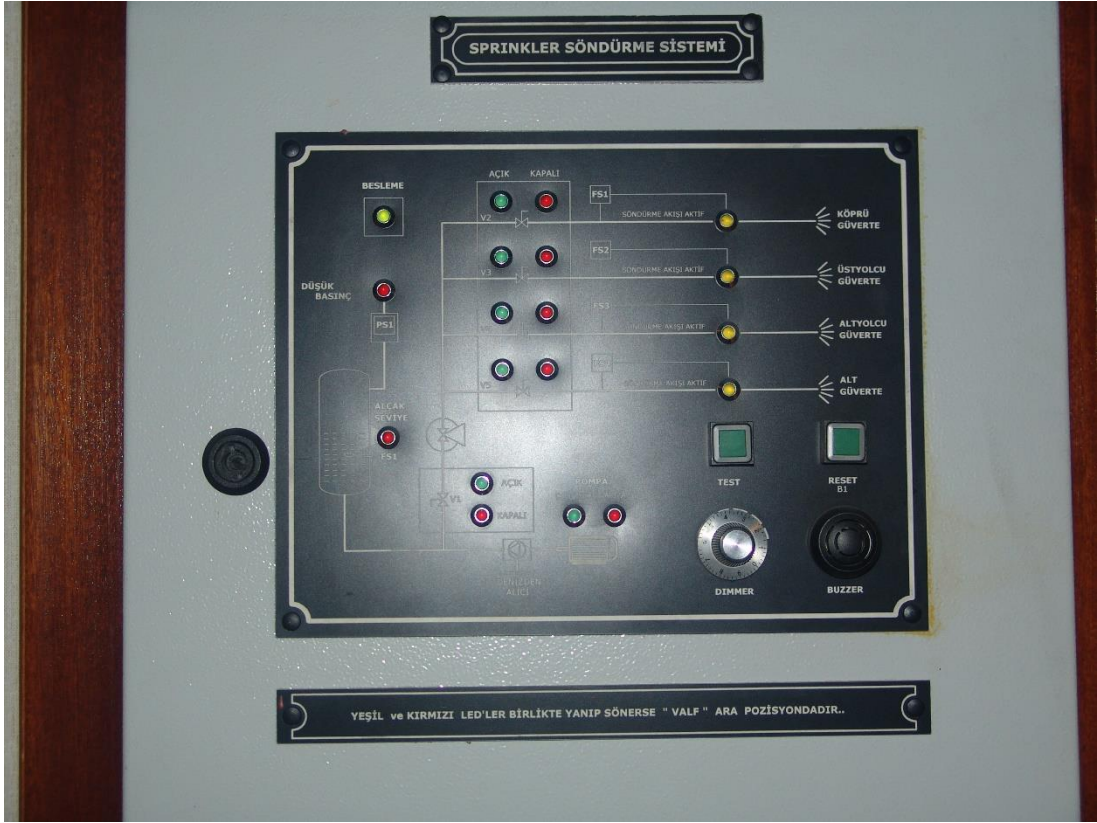
Figure A.15: Sprinkler Control System.
