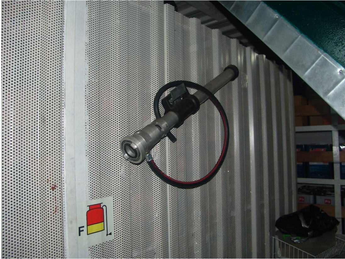
Figure A.7: Gun for Foam Making System.
